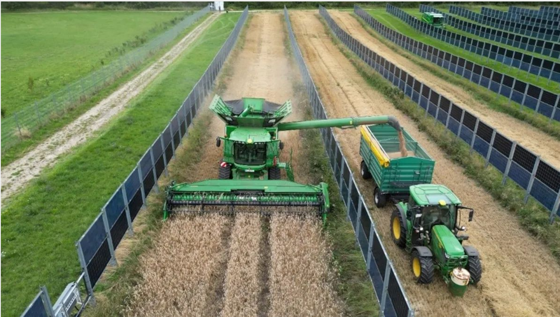
Next2Sun installs bifacial solar panels on its patented vertical mounting system (Electrek 2023)
